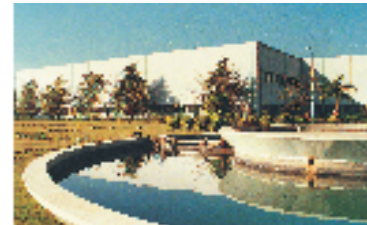
Switchgear Factory, Ahmednagar
