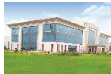
Switchgear Factory, Vadodara
