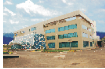
Switchgear Factory, Navi Mumbai
