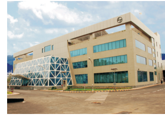
Switchgear Factory, Navi Mumbai
