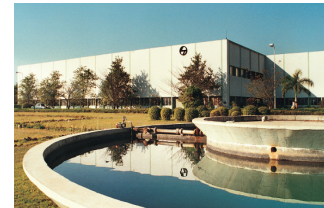
Switchgear Factory, Ahmednagar
