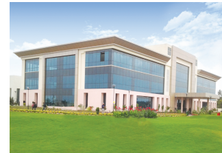
Switchgear Factory, Vadodara
