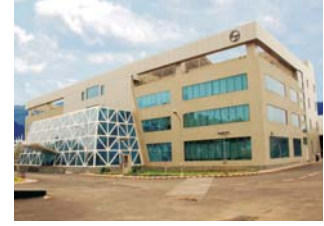
Switchgear Factory, Navi Mumbai
