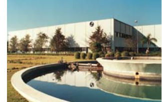
Switchgear Factory, Ahmednagar
