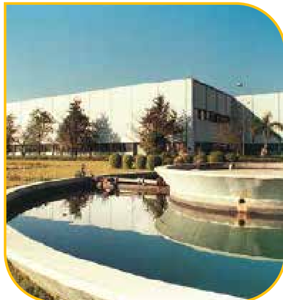
Switchgear Factory, Vadodara
