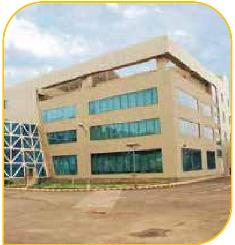
Switchgear Factory, Navi Mumbai
