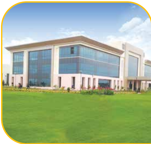
Switchgear Factory, Ahmednagar
