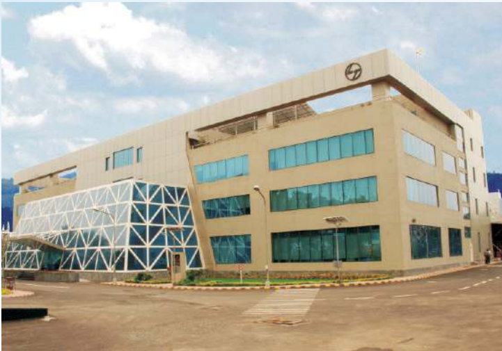
Switchgear Factory, Navi Mumbai
