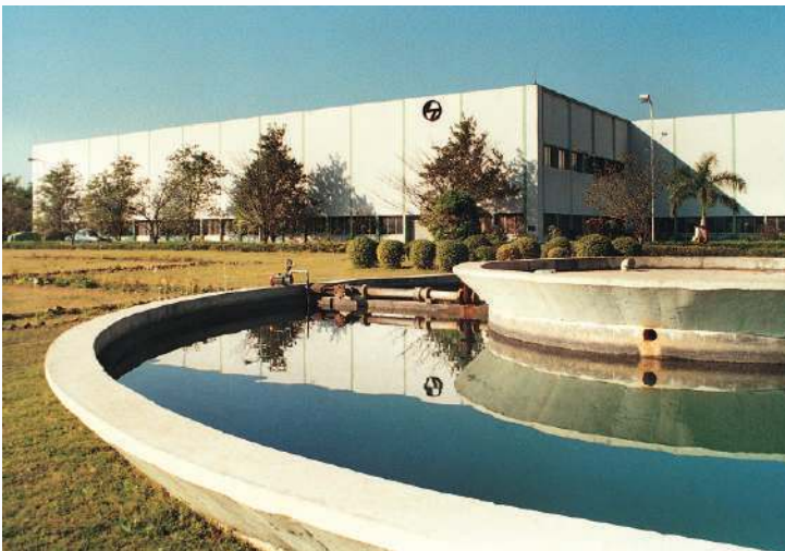
Switchgear Factory, Ahmednagar
