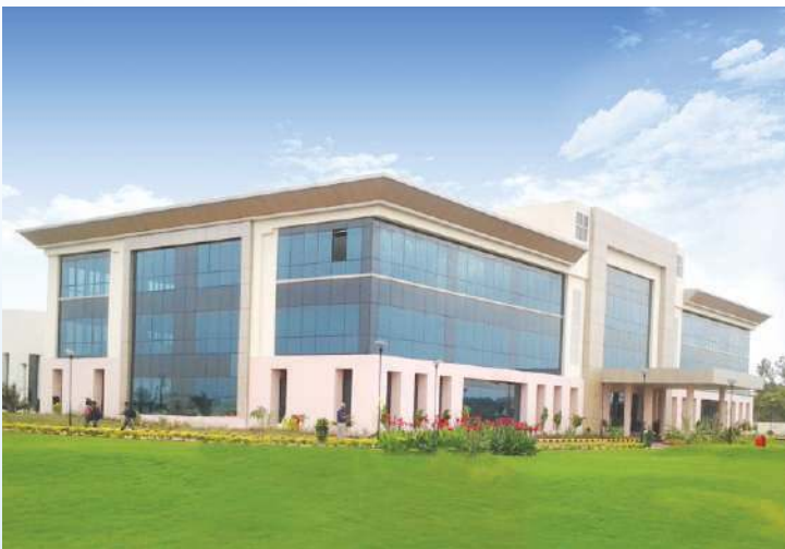
Switchgear Factory, Vadodara
