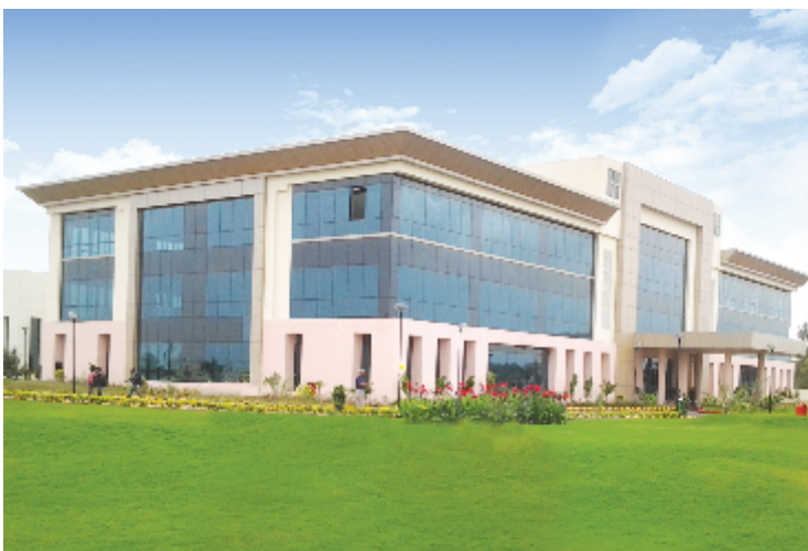
Switchgear Factory, Vadodara
