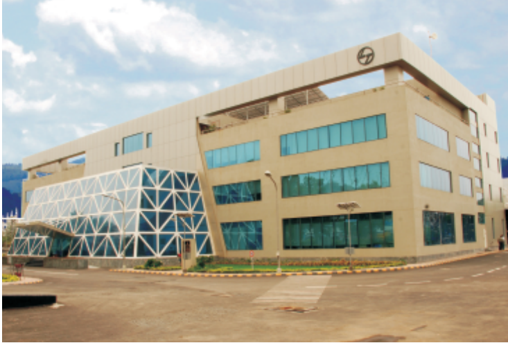
Switchgear Factory, Navi Mumbai
