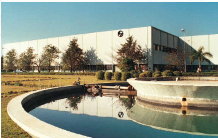
Switchgear Factory, Ahmednagar
