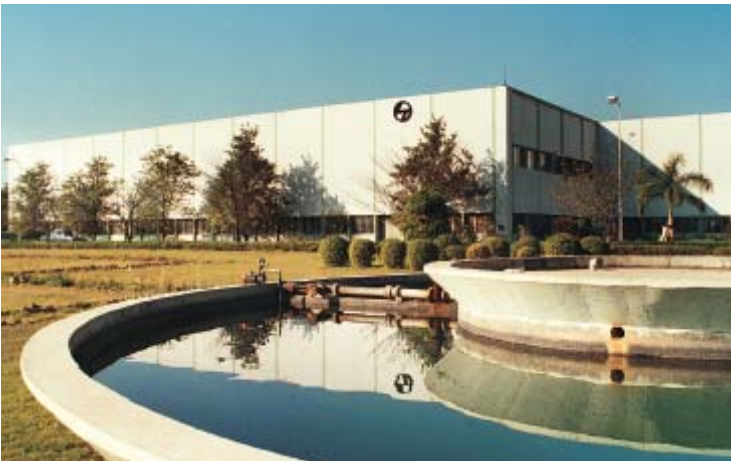
Switchgear Factory, Ahmednagar
