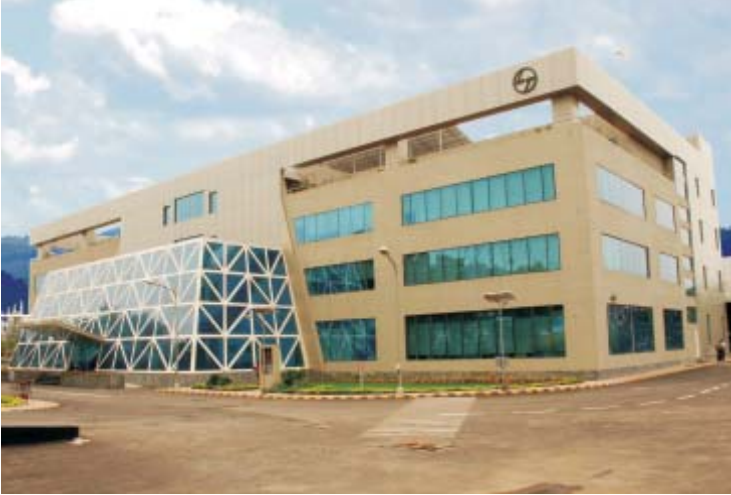
Switchgear Factory, Navi Mumbai
