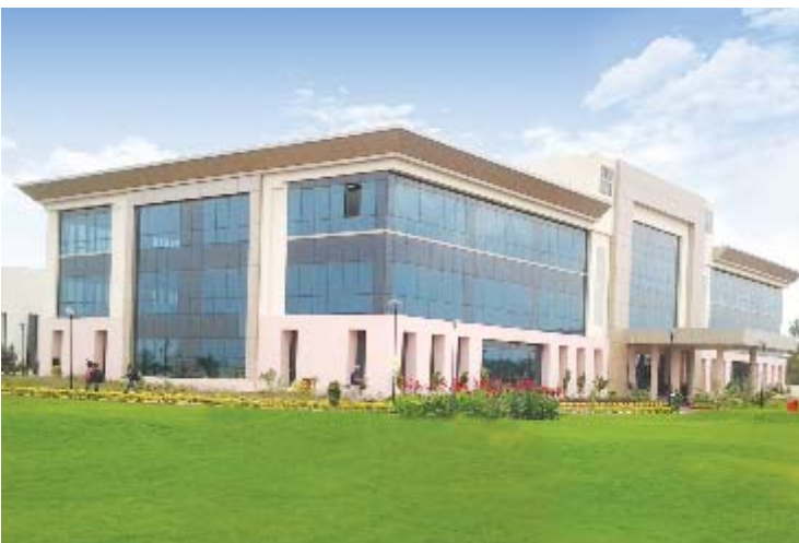
Switchgear Factory, Vadodara
