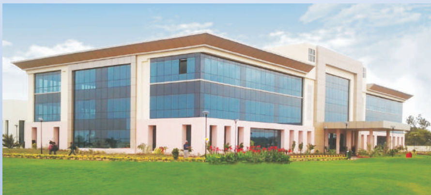
Switchgear Factory, Vadodara
