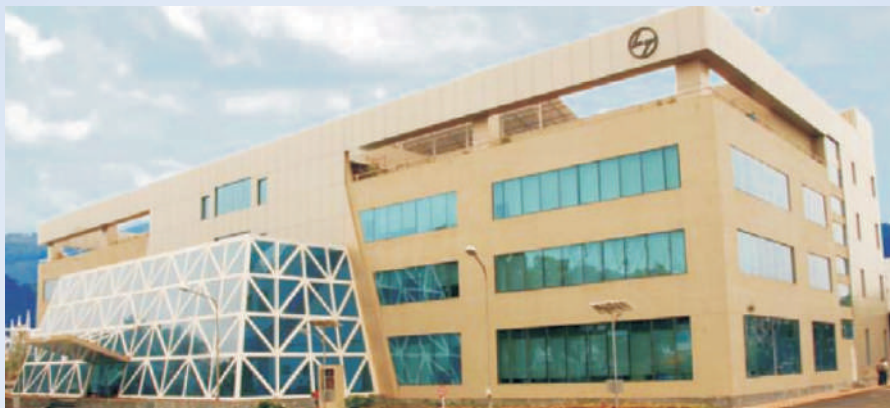
Switchgear Factory, Navi Mumbai
