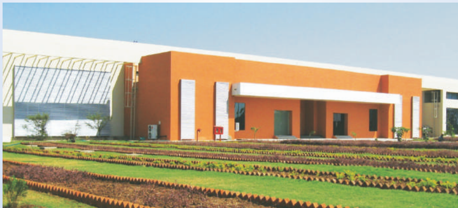
Switchgear Factory, Ahmednagar
