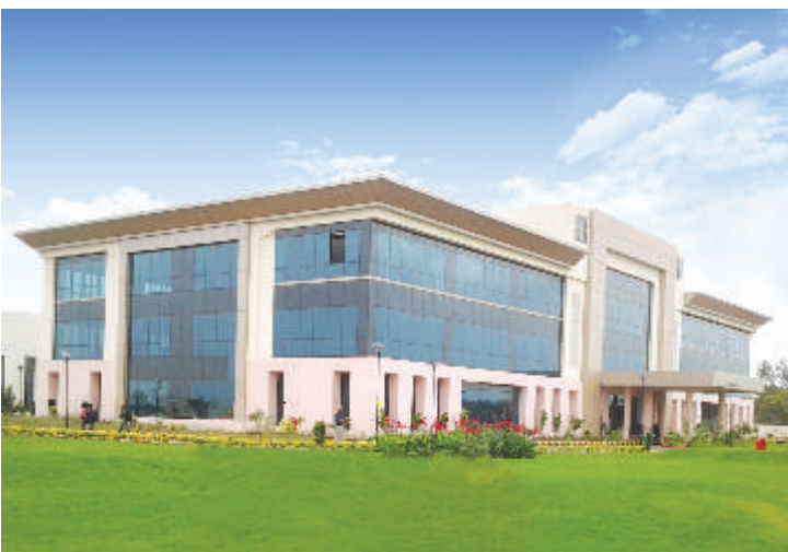
Switchgear Factory, Vadodara
