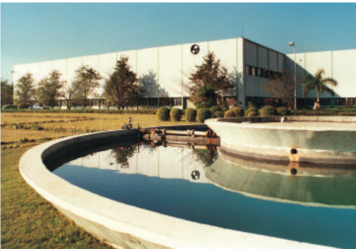
Switchgear Factory, Ahmednagar
