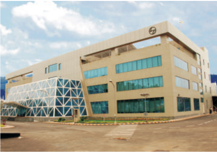
Switchgear Factory, Navi Mumbai
