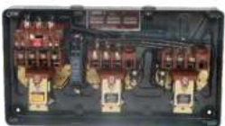
Interior View of MK2 FASD
