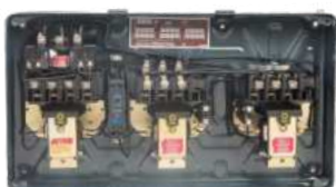
Interior View of MK1 FASD
