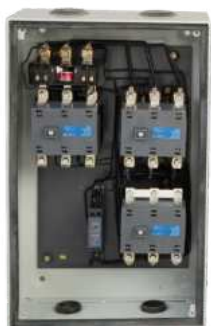
Interior View of ML FASD
